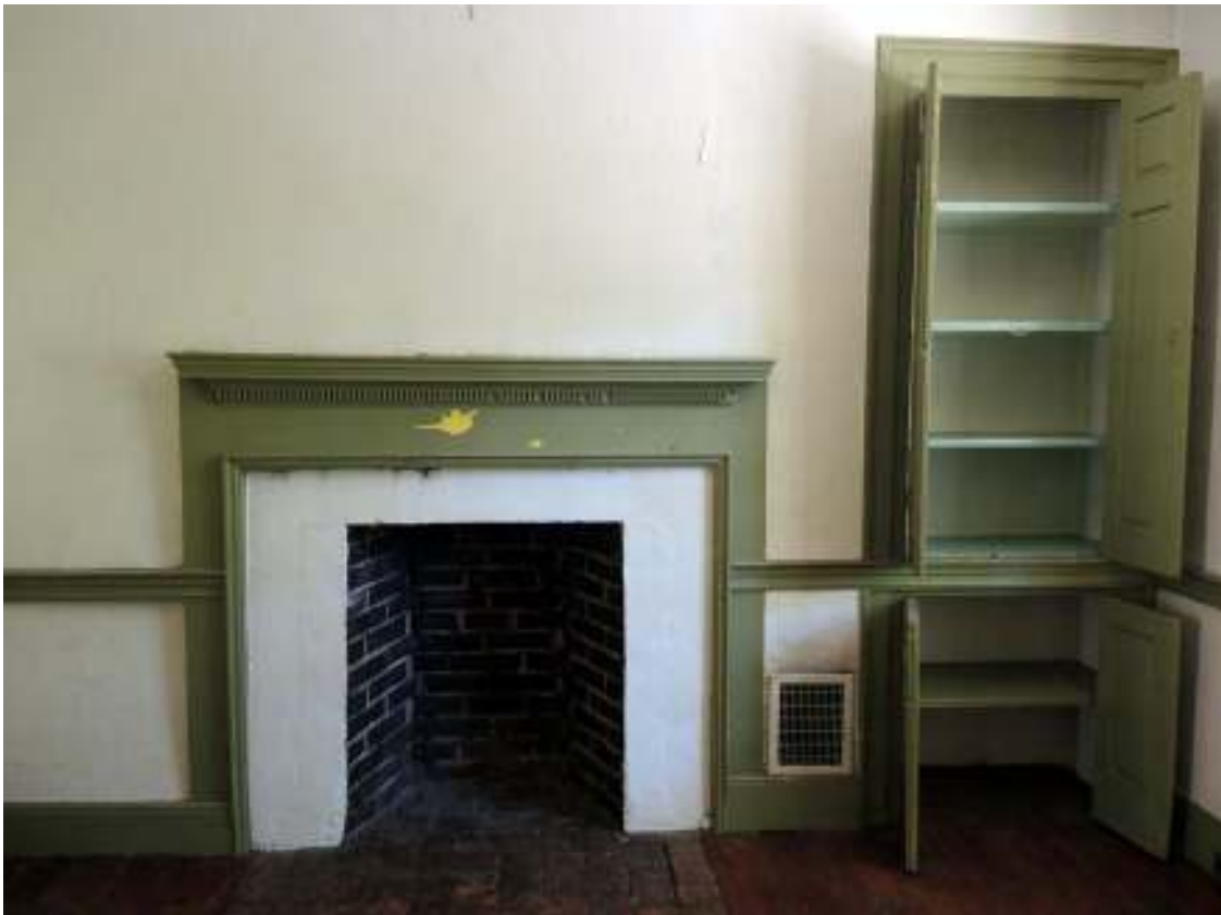
PHOTO 143 - Ell Interior, Room 208, South Wall (09-14-2016, NTHP)
