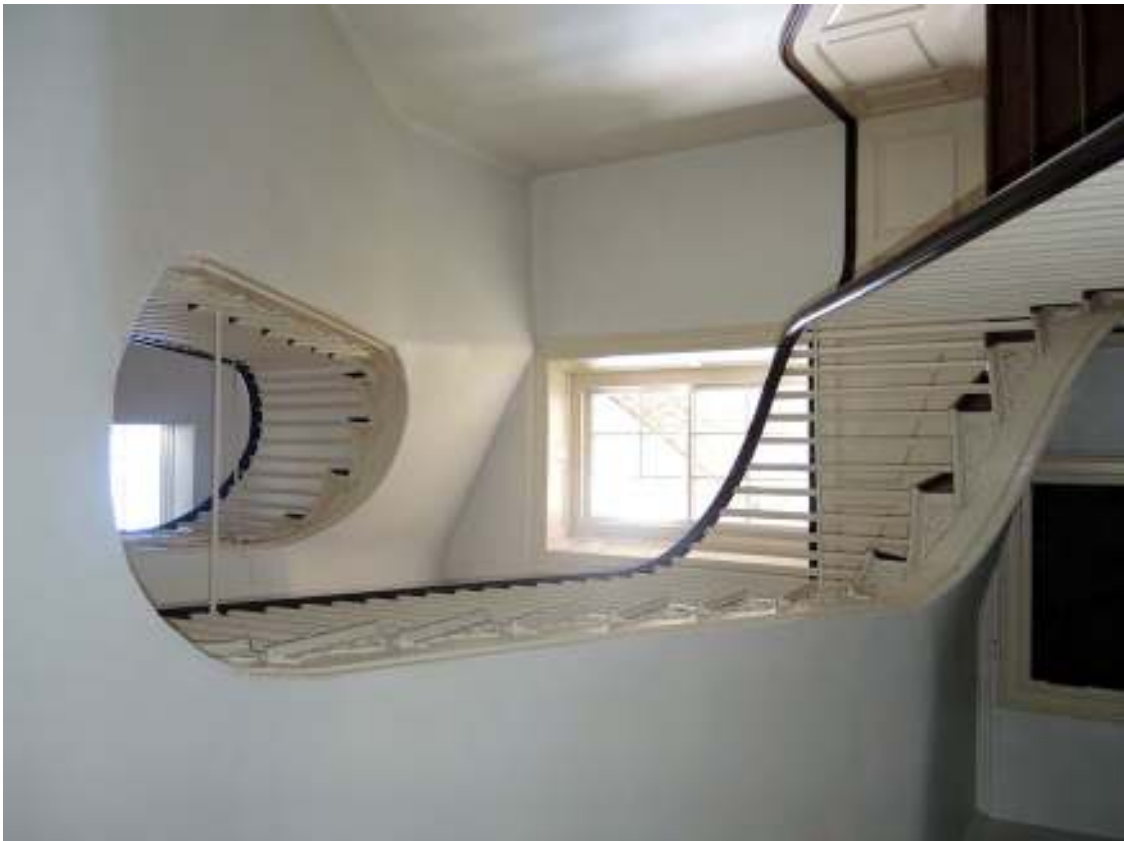
PHOTO 052 - Main Block Interior, Room 102, Looking Southwest (09-13-2016, NTHP)
