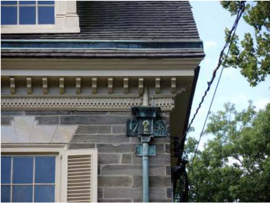
PHOTO 045 - Main Block, Detail of Northwest Corner (09-13-2016, NTHP)
