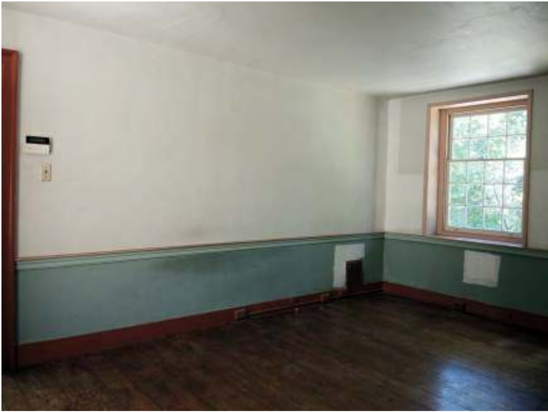
PHOTO 132 - Ell Interior, Room 206, Southwest Corner (09-14-2016, NTHP)
