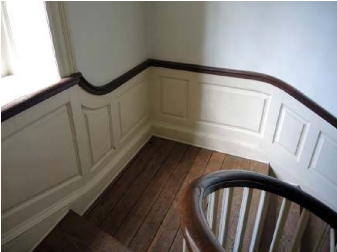
PHOTO 102 - Main Block Interior, Room 202, Looking Northwest (09-13-2016, NTHP)
