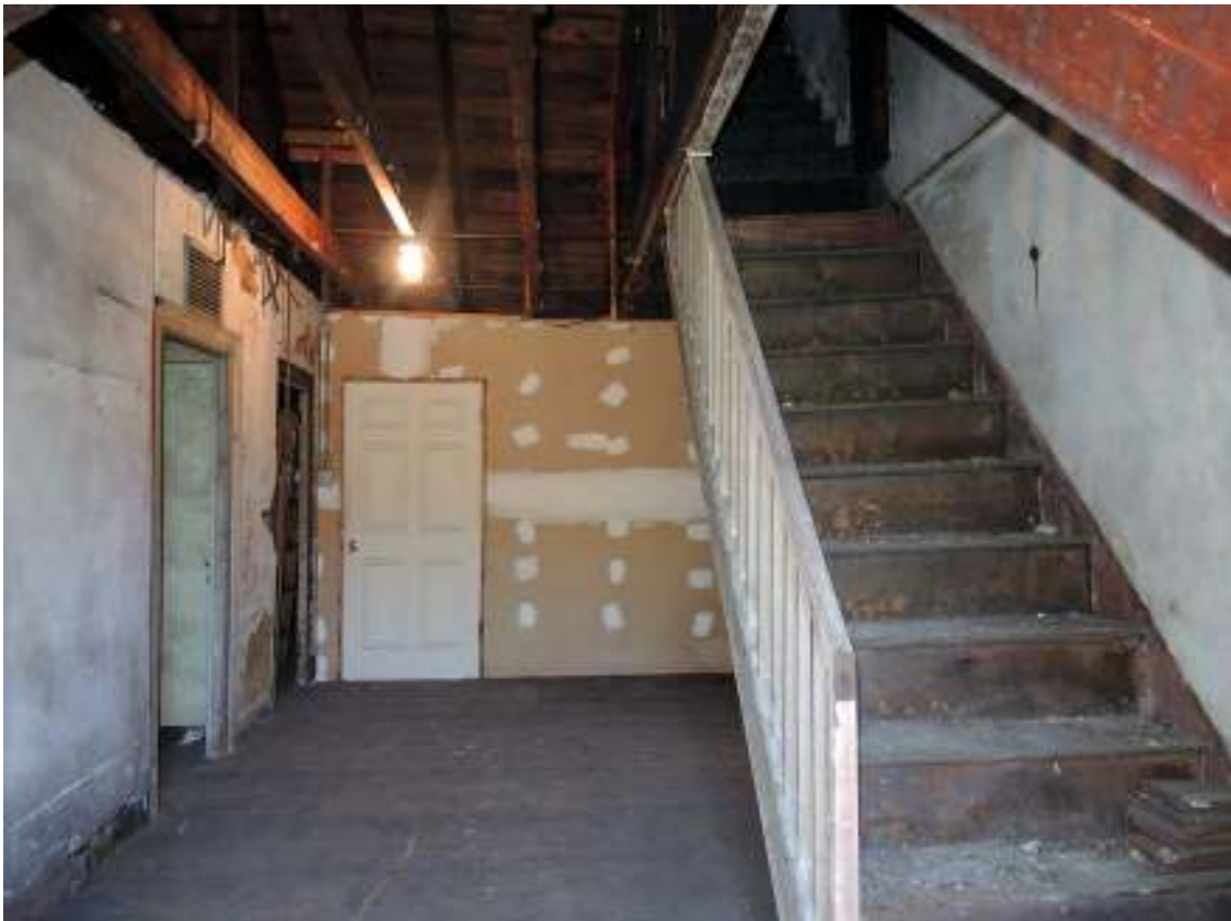
PHOTO 161 - Main Block Interior, Room 302, Looking Southwest (09-14-2016, NTHP)
