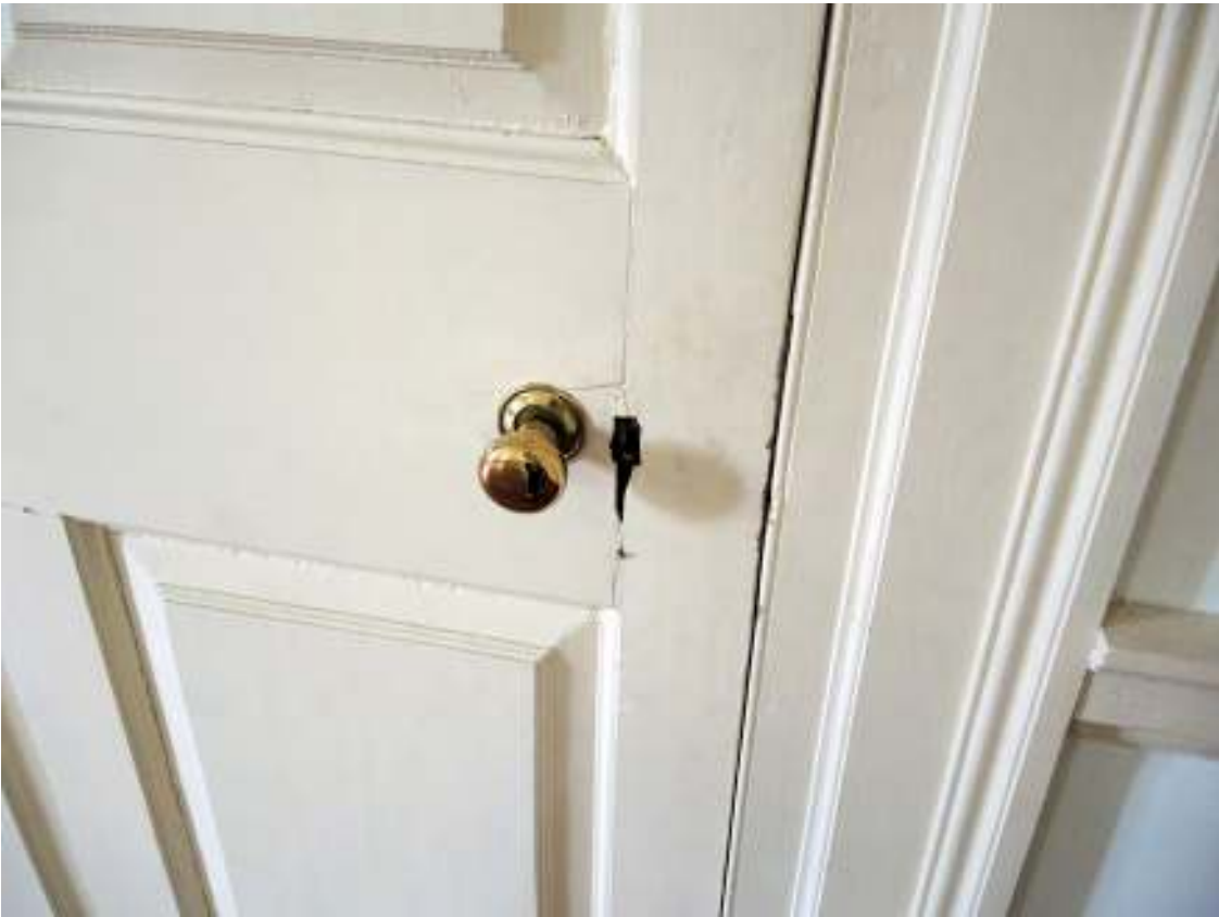
PHOTO 121 - Main Block Interior, Room 204, Detail of Closet Hardware (09-13-2016, NTHP)
