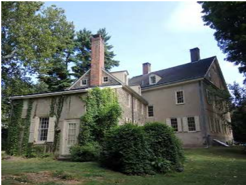
PHOTO 023 - Rear Extension, Ell, and Main Block, South Elevation (09-13-2016, NTHP)
