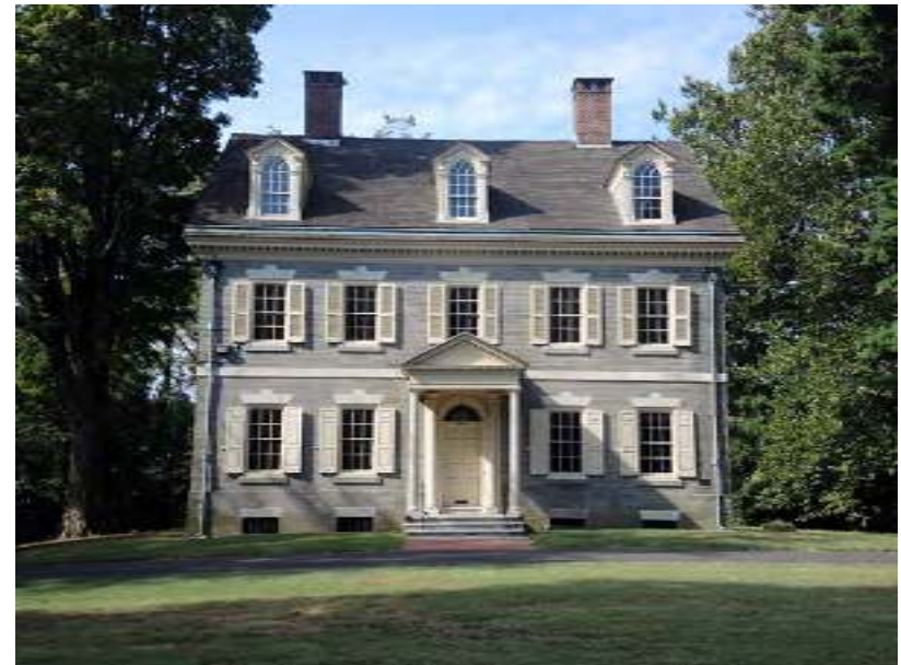
PHOTO 040 - Main Block, North Facade (09-13-2016, NTHP)
