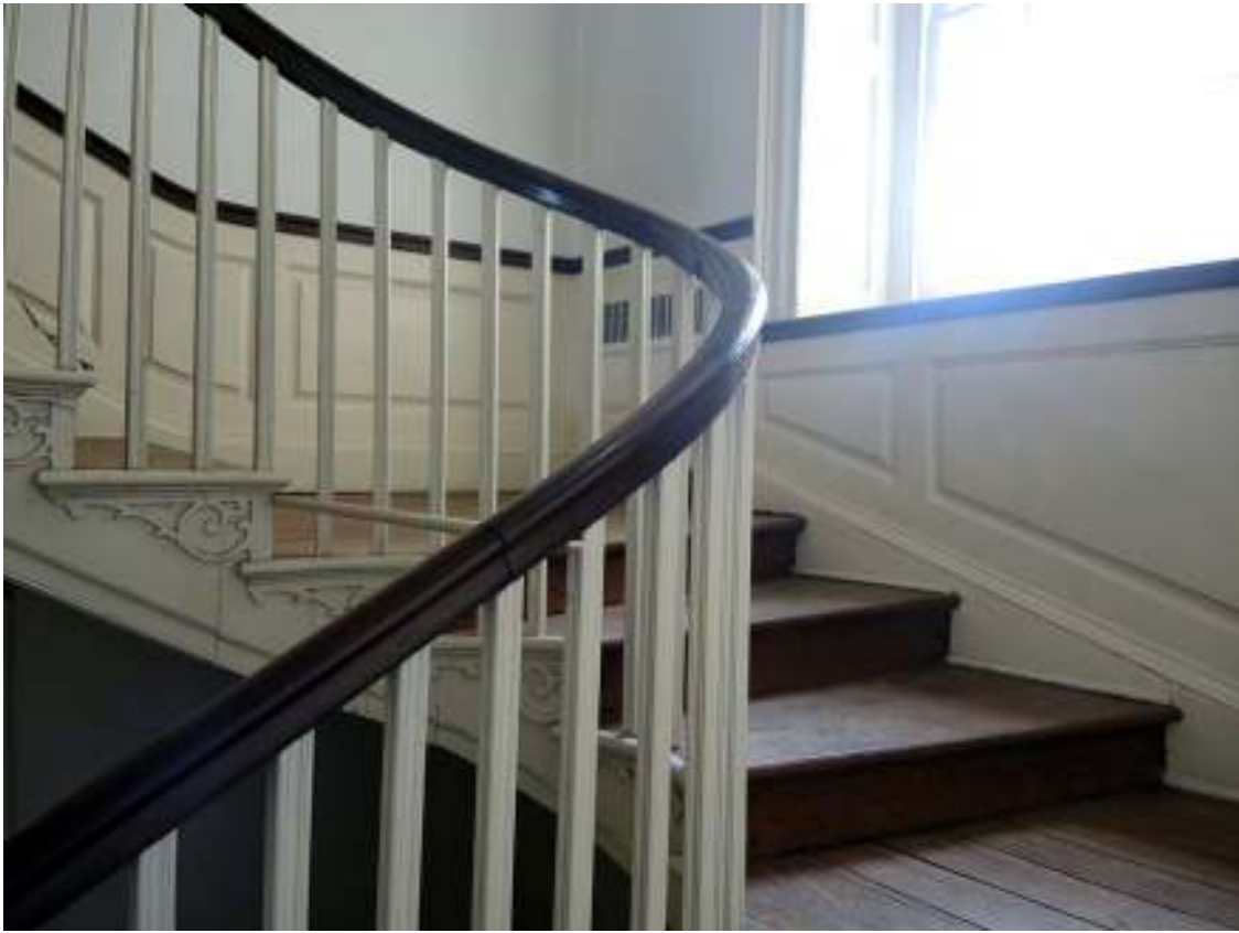
PHOTO 101 - Main Block Interior, Room 202, Looking Southeast (09-13-2016, NTHP)
