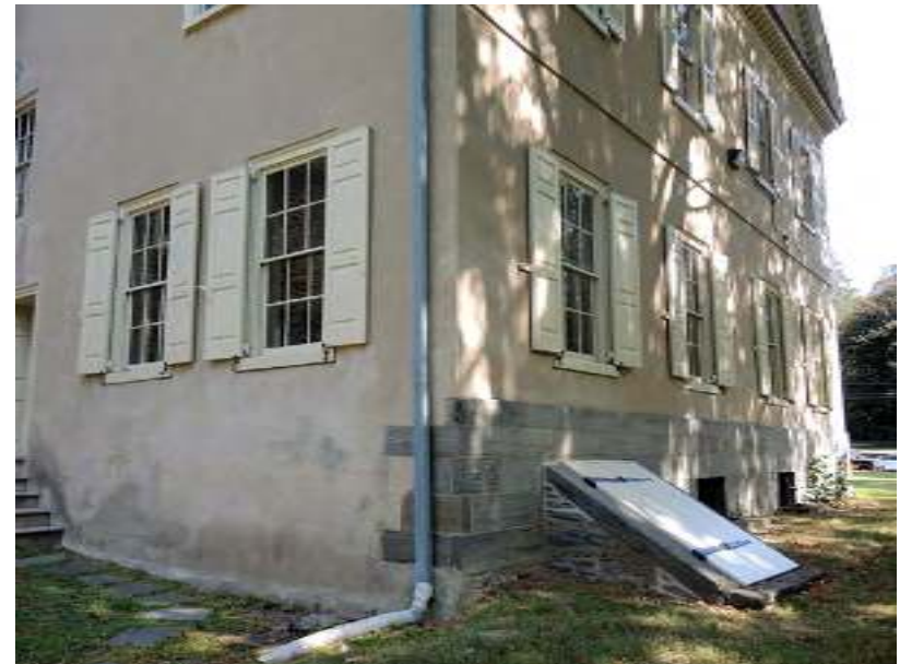
PHOTO 028 - Main Block, Southeast Corner (09-13-2016, NTHP)
