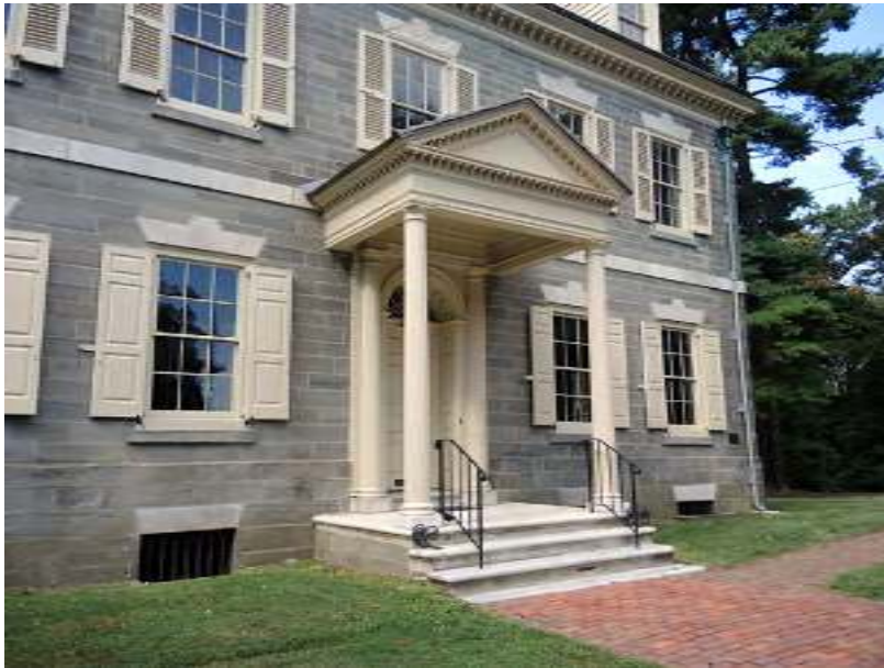
PHOTO 037 - Main Block, North Facade (09-13-2016, NTHP)
