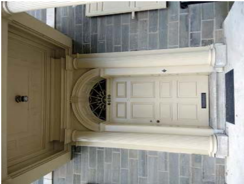
PHOTO 043 - Main Block, North Facade, Detail of Entry Door and Portico (09-13-2016, NTHP)
