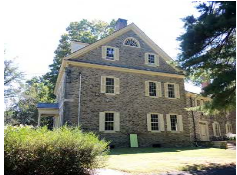
PHOTO 012 - Main Block, West Elevation (09-14-2016, NTHP)
