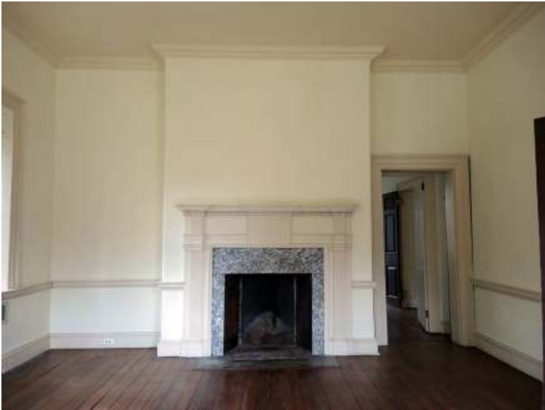
PHOTO 105 - Main Block Interior Room 201, South Wall (09-13-2016, NTHP)
