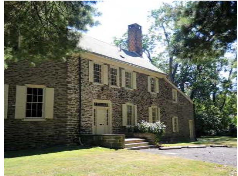
PHOTO 014 - Ell and Rear Extension, West Elevation (09-14-2016, NTHP)
