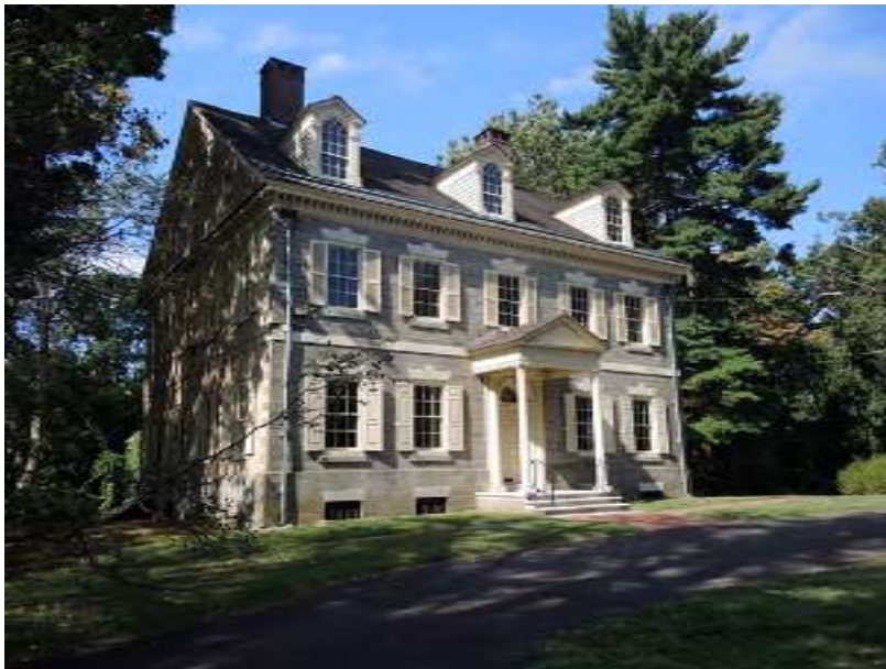
PHOTO 039 - Main Block, Northeast Corner (09-13-2016, NTHP)
