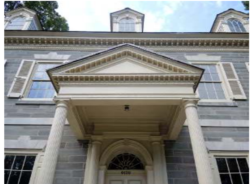
PHOTO 042 - Main Block, North Facade (09-13-2016, NTHP)
