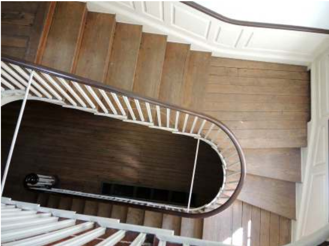
PHOTO 157 - Main Block Interior, Room 302, Looking Down (09-14-2016, NTHP)
