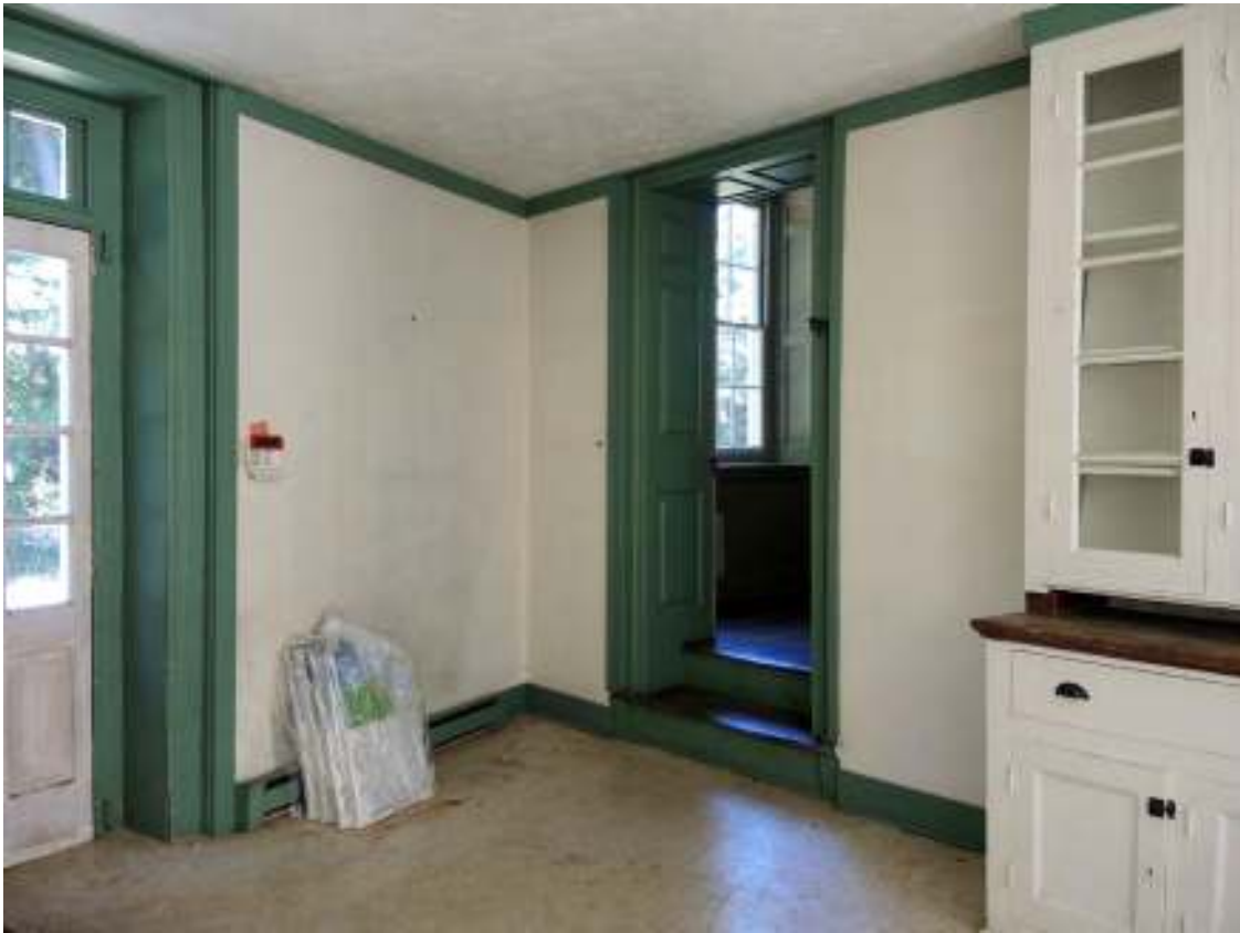
PHOTO 087 - Ell Interior, Room 106, Northwest Corner (09-14-2016, NTHP)
