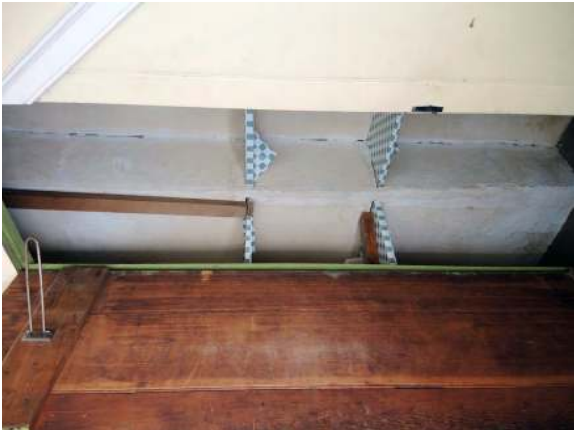
PHOTO 147 - Ell Interior, Room 209, Detail of Closet Below Stair (09-14-2016, NTHP)
