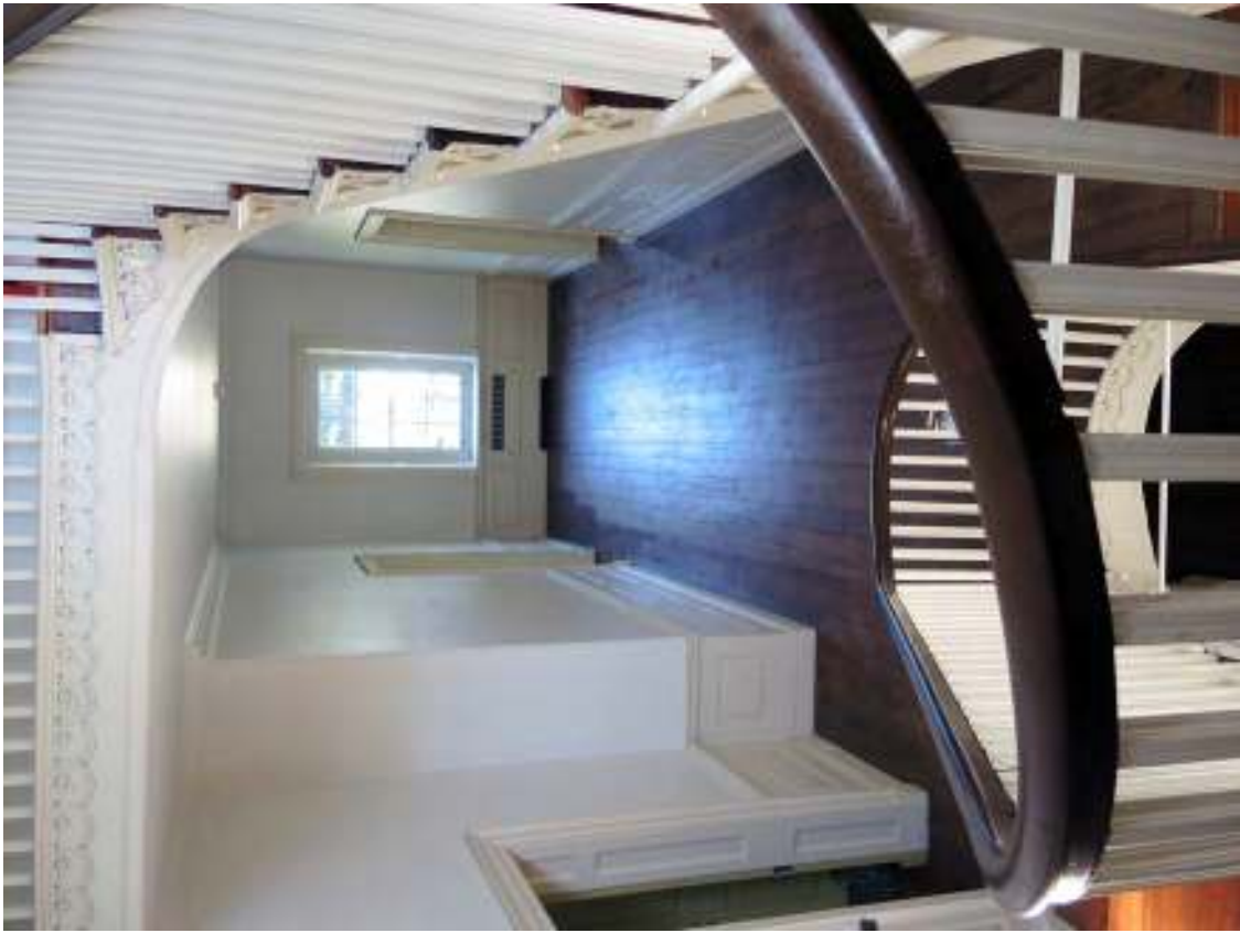
PHOTO 156 - Main Block Interior, Room 302, Looking Northeast (09-14-2016, NTHP)
