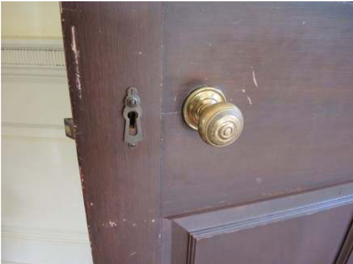
PHOTO 062 - Main Block Interior, Room 101, Detail of Door Hardware (09-13-2016, NTHP)
