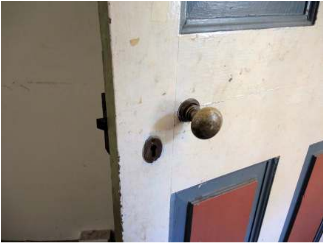
PHOTO 142 - Ell Interior, Room 208, Detail of Door Hardware (09-14-2016, NTHP)
