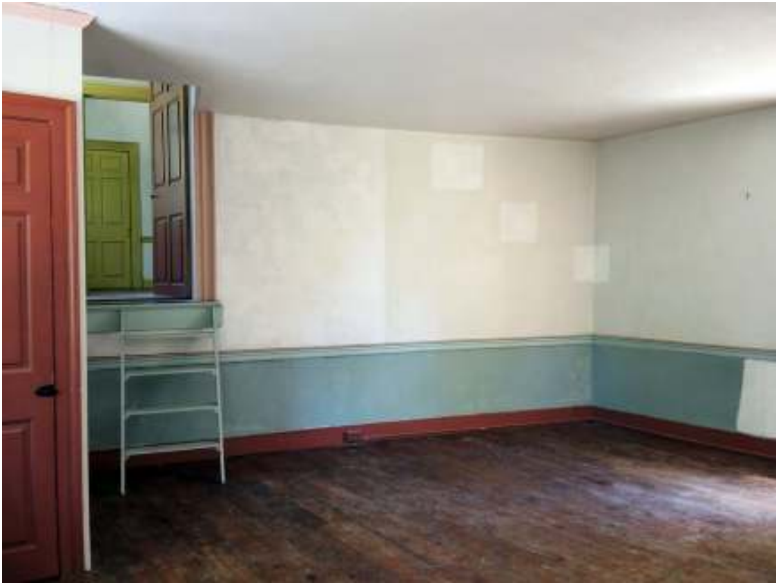
PHOTO 134 - Ell Interior, Room 206, Northeast Corner (09-14-2016, NTHP)
