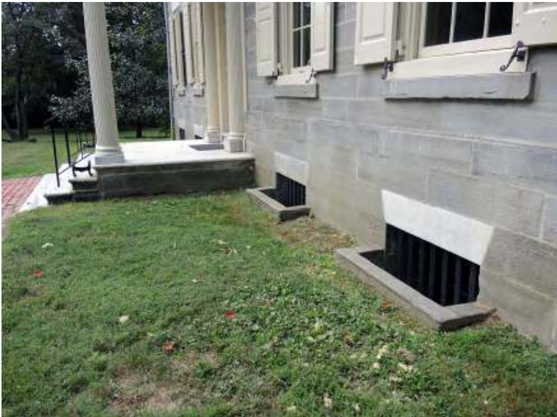
PHOTO 046 - Main Block, North Facade, Looking Southeast (09-13-2016, NTHP)
