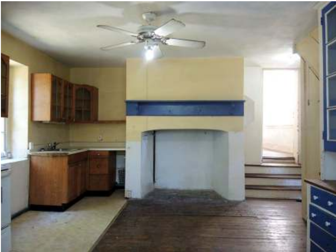
PHOTO 096 - Rear Extension Interior, Room 108, North Wall (09-14-2016, NTHP)
