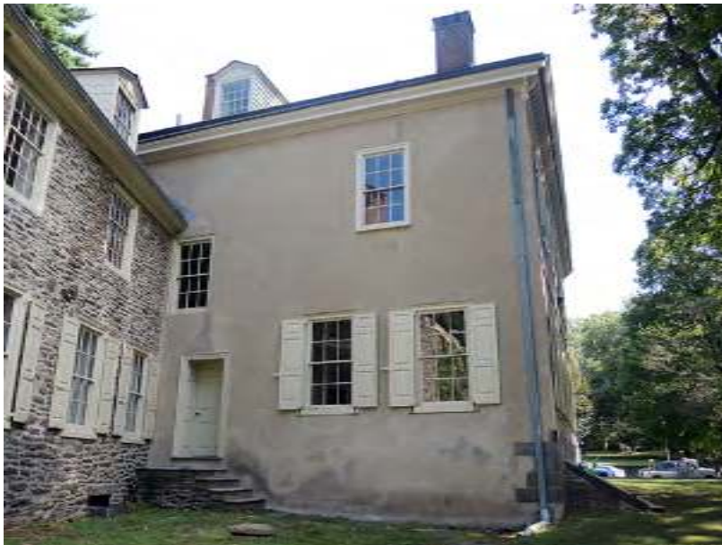
PHOTO 027 - Main Block, South Elevation (09-13-2016, NTHP)
