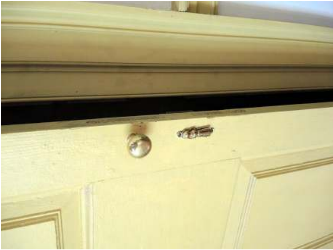
PHOTO 126 - Main Block Interior, Room 205, Detail of Closet Hardware (09-13-2016, NTHP)
