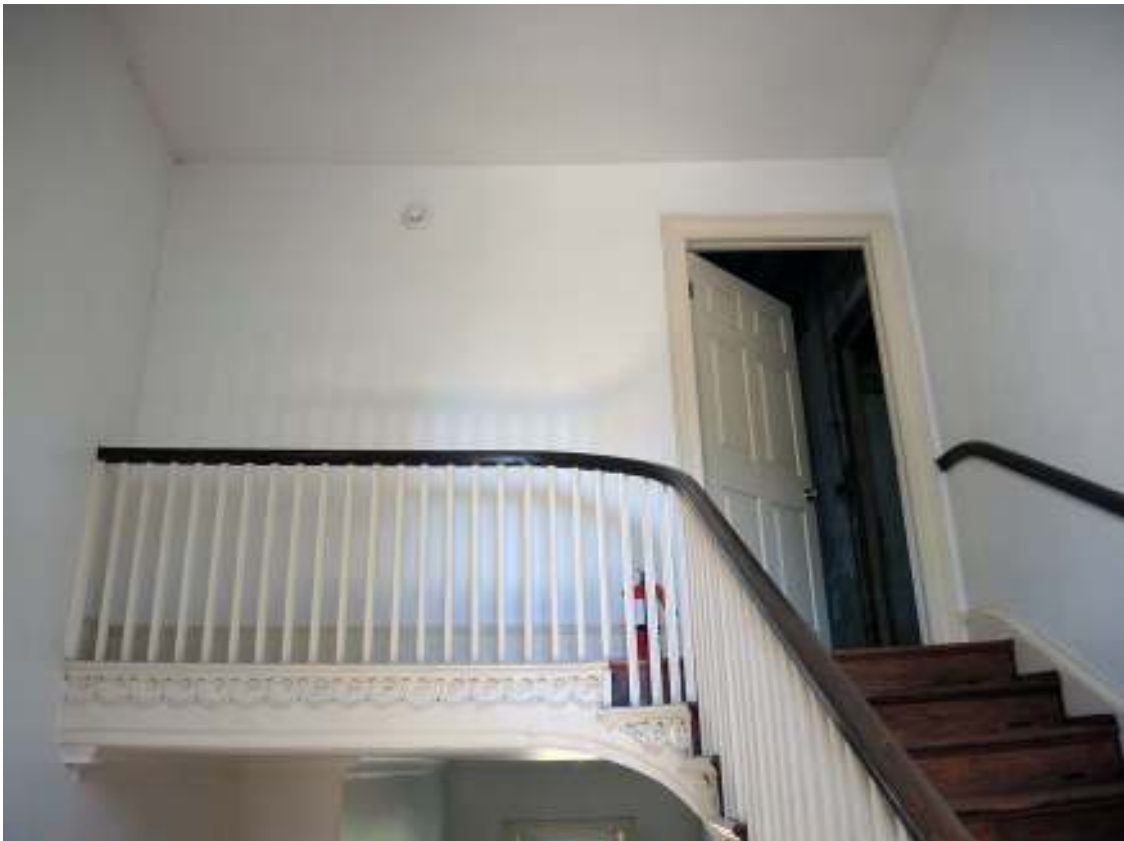
PHOTO 159 - Main Block Interior, Room 302, Looking Northeast (09-14-2016, NTHP)
