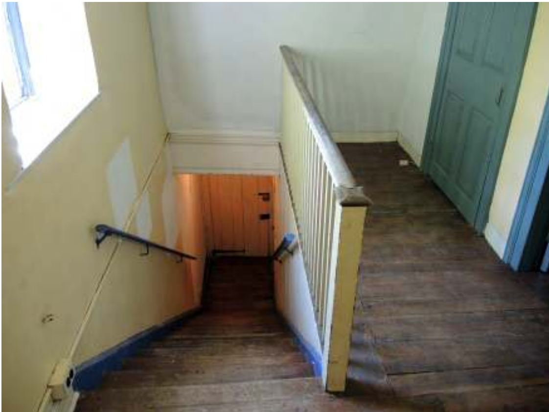
PHOTO 149 - Rear Extension Interior, Room 209, Looking Southwest (09-14-2016, NTHP)
