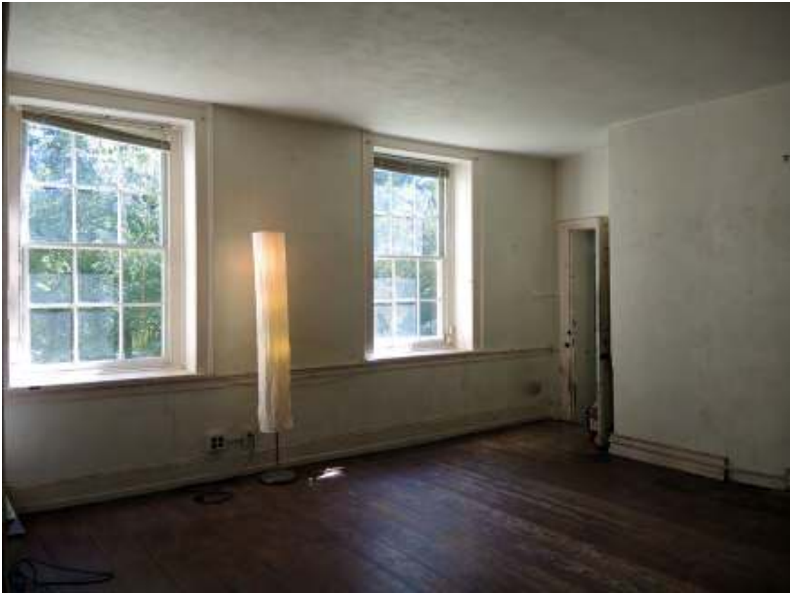
PHOTO 089 - Ell Interior, Room 107, Southeast Corner (09-14-2016, NTHP)
