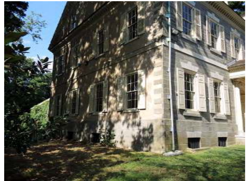
PHOTO 036 - Main Block, Northeast Corner (09-13-2016, NTHP)
