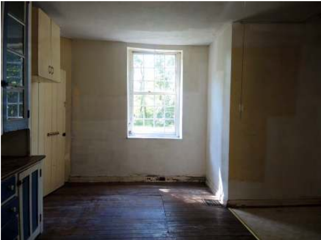
PHOTO 094 - Rear Extension Interior, Room 108, South Wall (09-14-2016, NTHP)
