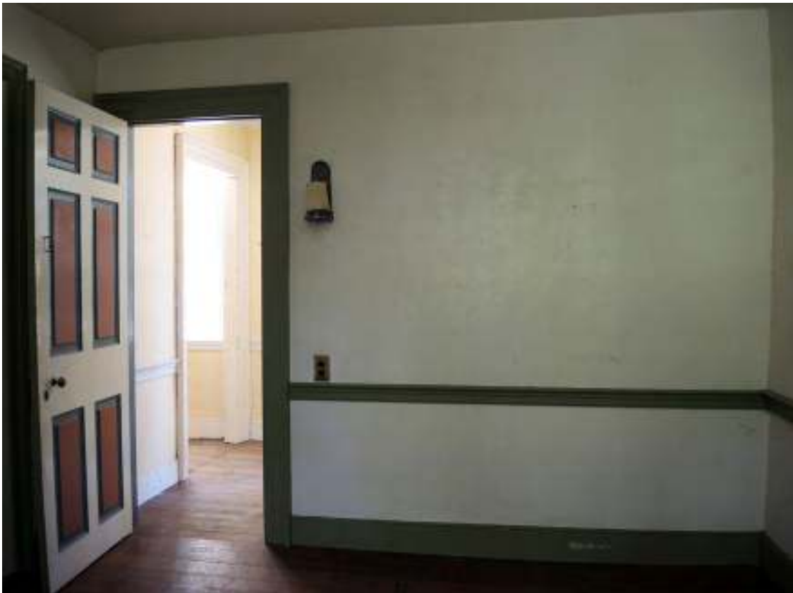
PHOTO 141 - EII Interior, Room 208, East Wall (09-14-2016, NTHP)
