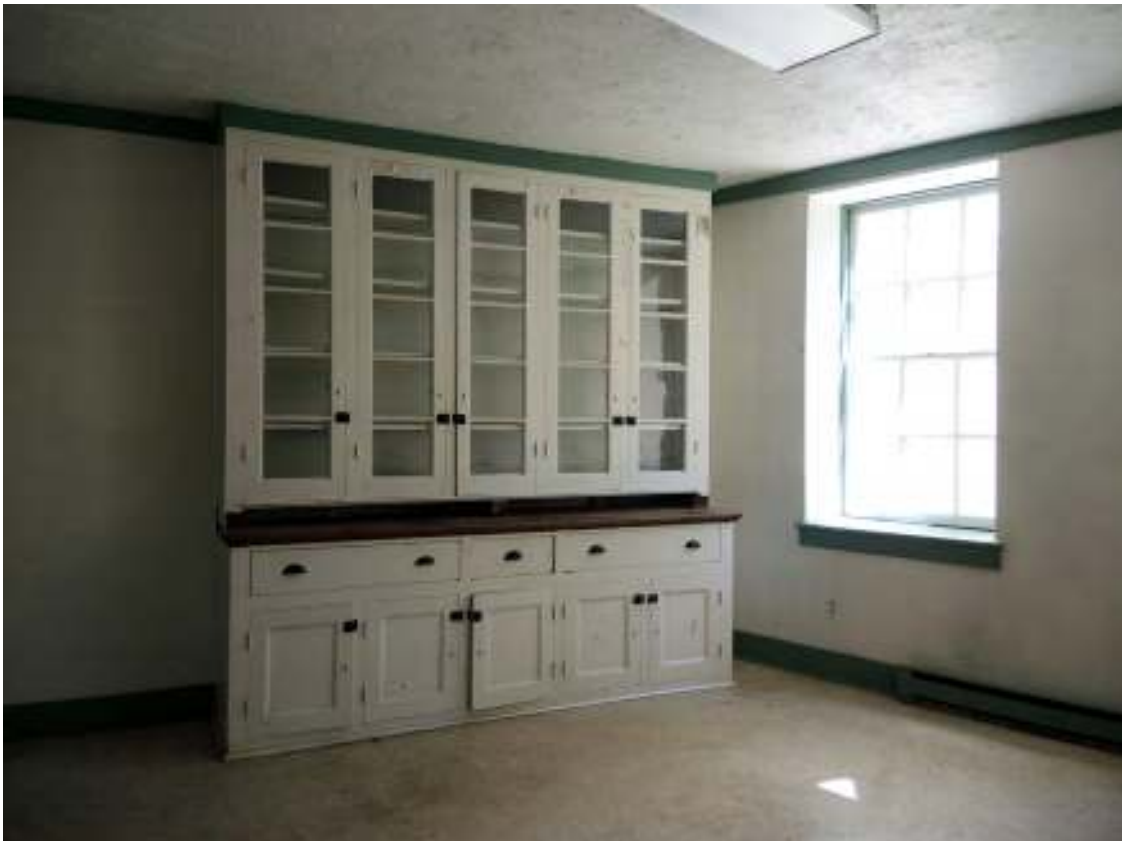
PHOTO 088 - Ell Interior, Room 106, Northeast Corner (09-14-2016, NTHP)
