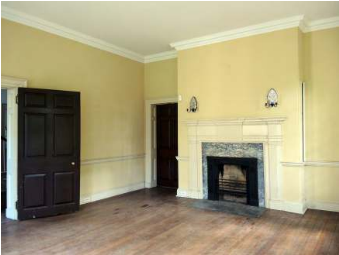
PHOTO 077 - Main Block Interior, Room 104, Northwest Corner (09-13-2016, NTHP)
