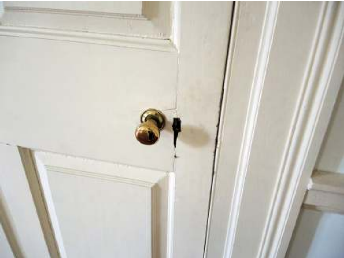
PHOTO 121 - Main Block Interior, Room 204, Detail of West Door Hardware (09-13-2016, NTHP)
