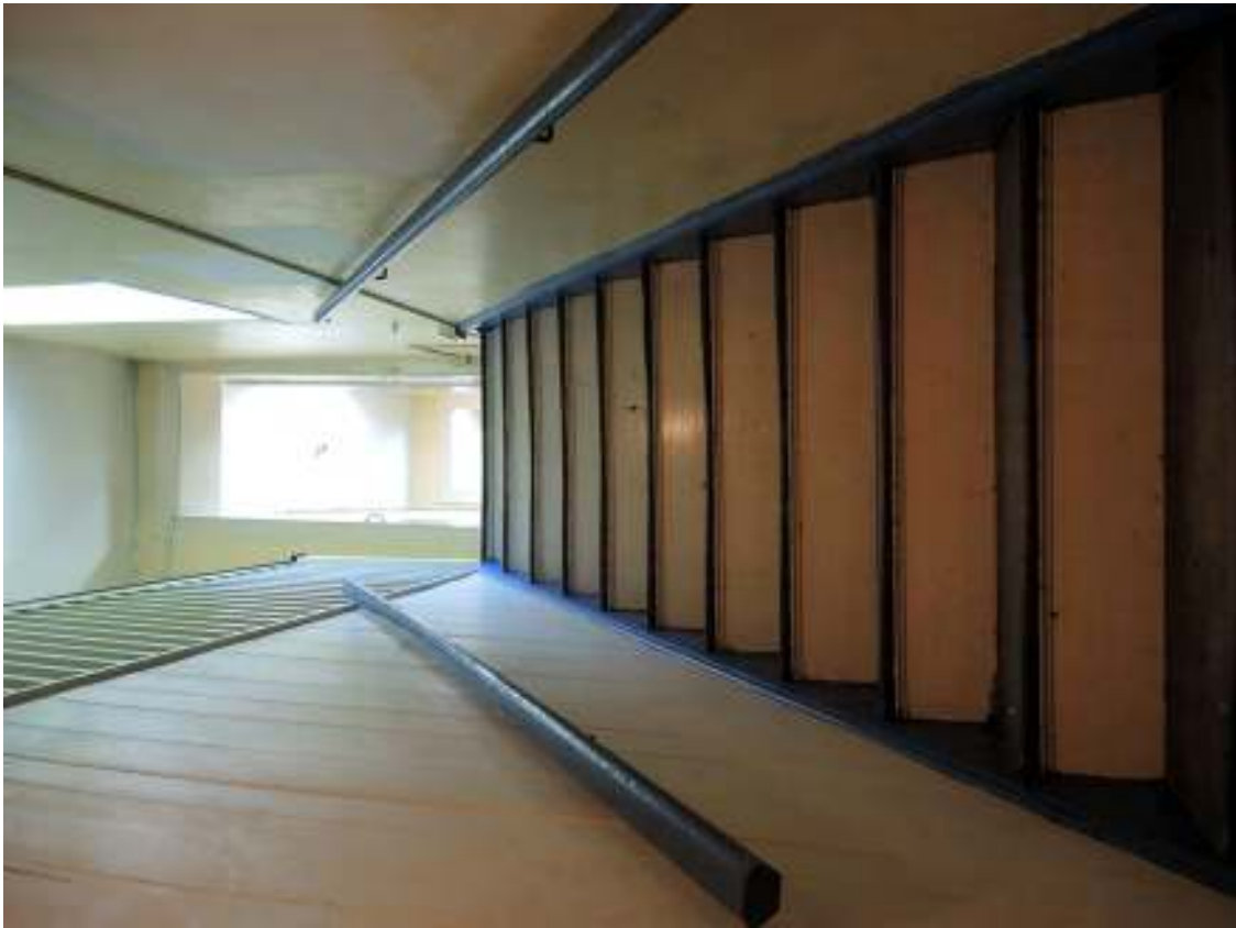
PHOTO 099 - Rear Extension Interior, Room 109, Looking Northeast (09-14-2016, NTHP)
