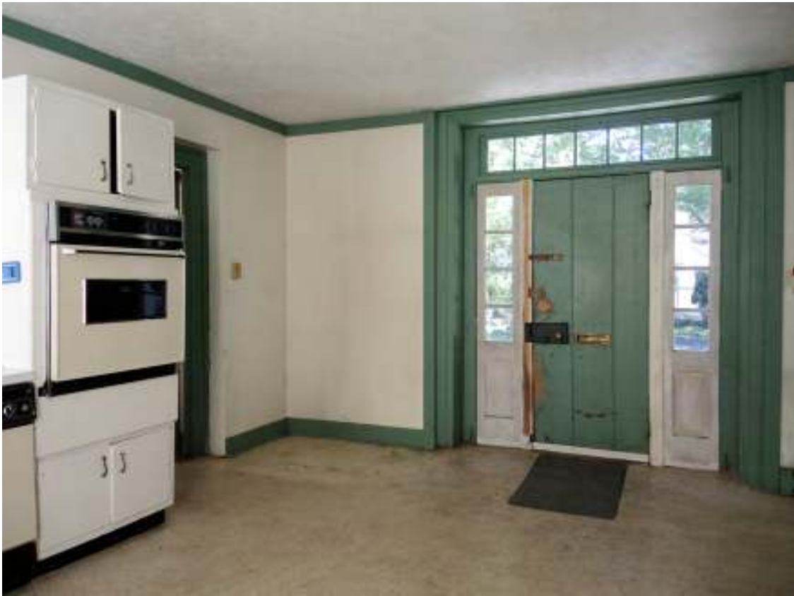
PHOTO 085 - Ell Interior, Room 106, Southwest Corner (09-14-2016, NTHP)
