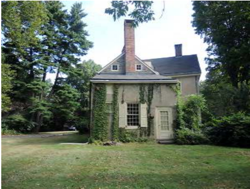
PHOTO 021 - Rear Extension, South Elevation (09-13-2016, NTHP)
