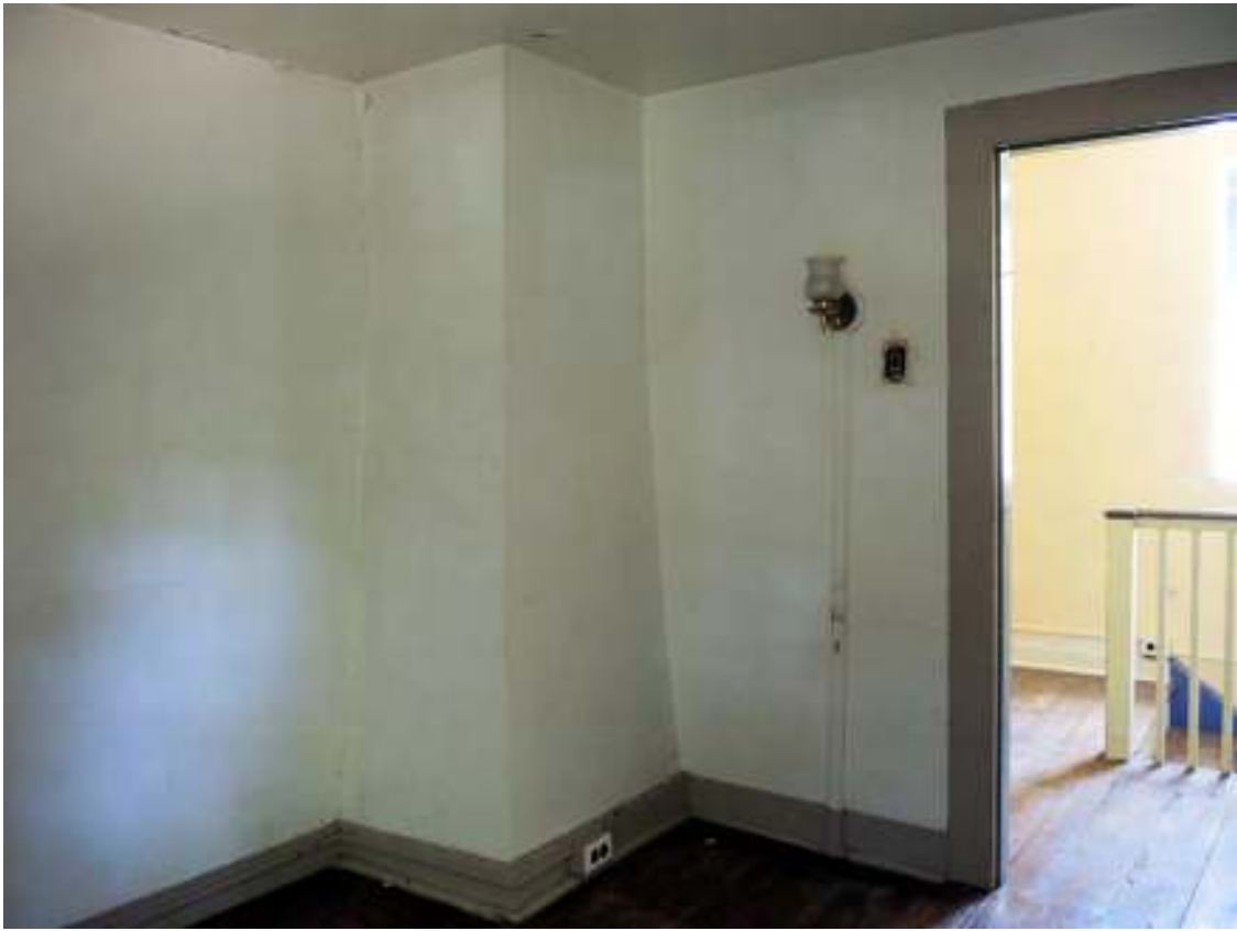
PHOTO 152 - Rear Extension Interior, Room 210, Northeast Corner (09-14-2016, NTHP)
