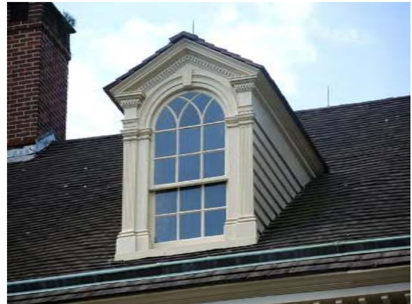
PHOTO 044 - Main Block, North Facade, Detail of Dormer Window (09-13-2016, NTHP)
