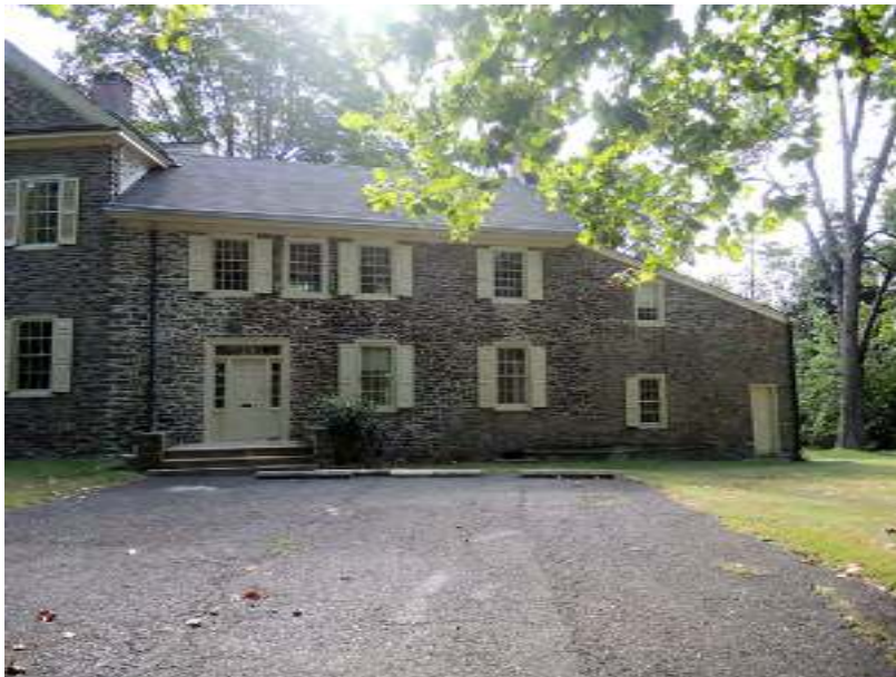
PHOTO 015 - Ell and Rear Extension, West Elevation (09-13-2016, NTHP)
