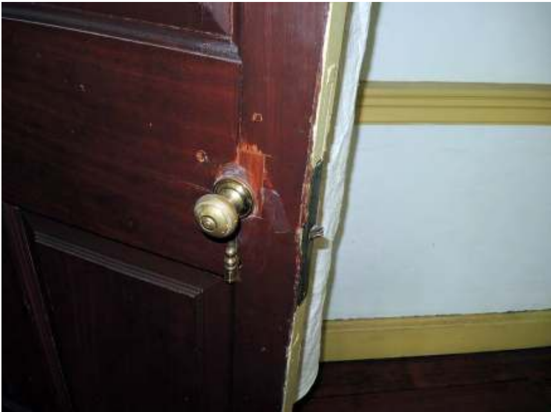
PHOTO 123 - Main Block Interior, Room 205, Detail of Door Hardware (09-13-2016, NTHP)
