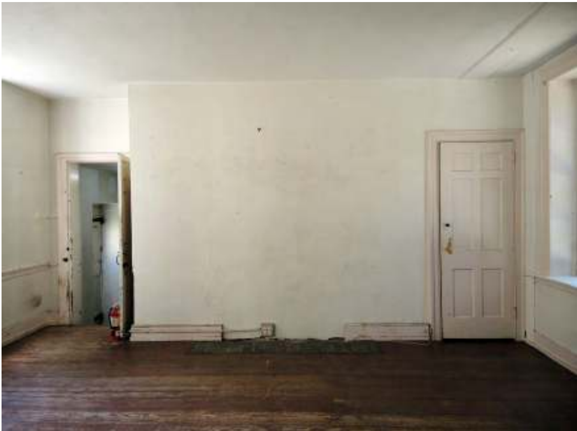
PHOTO 090 - Ell Interior, Room 107, South Wall (09-14-2016, NTHP)
