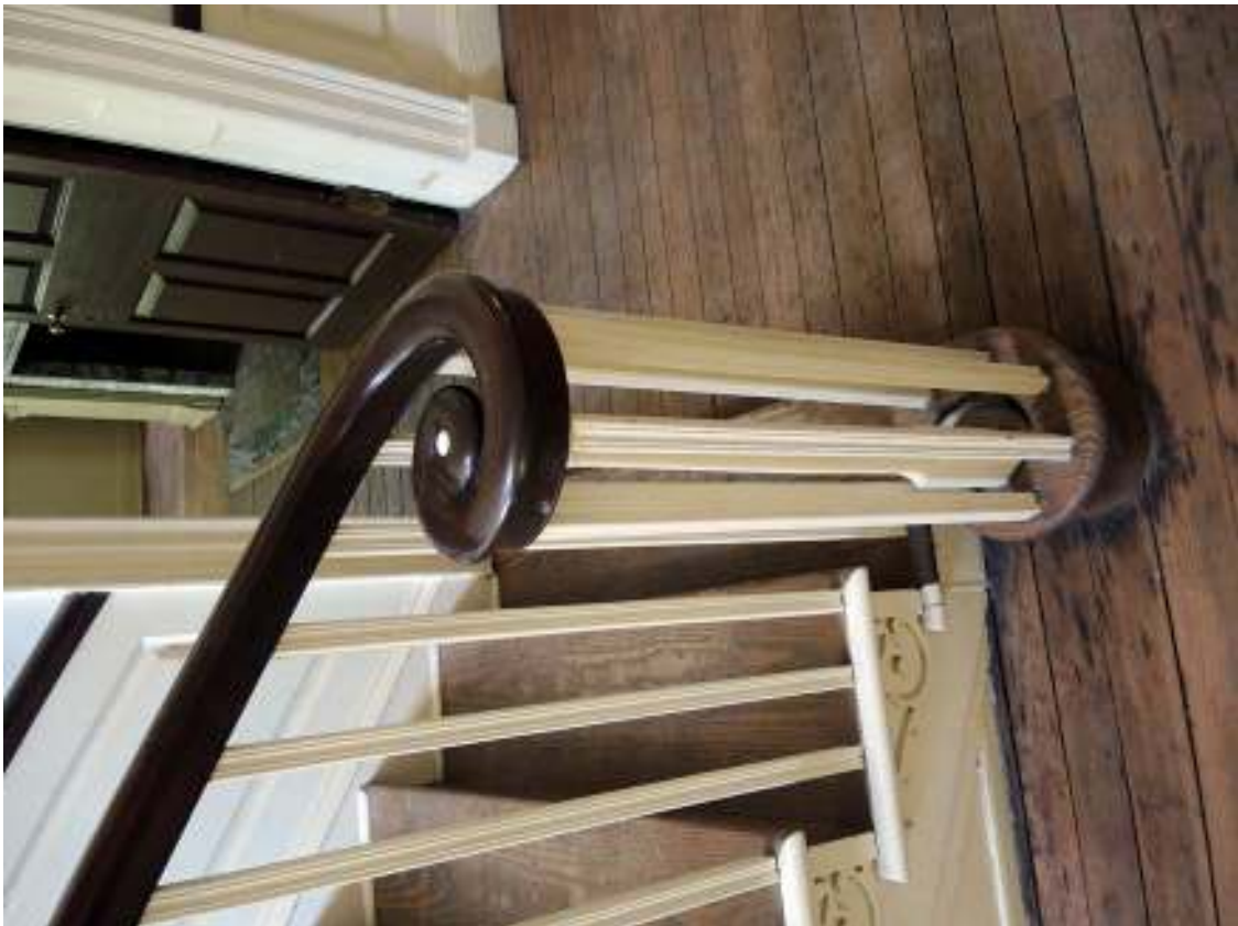
PHOTO 050 - Main Block Interior, Room 102, Detail of Newel and Handrail (09-13-2016, NTHP)
