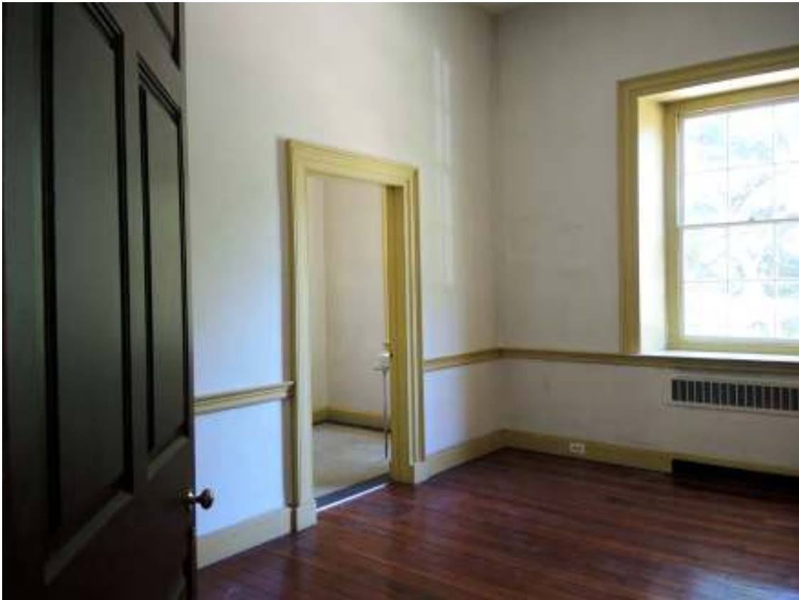
PHOTO 122 - Main Block Interior, Room 205, Southwest Corner (09-14-2016, NTHP)
