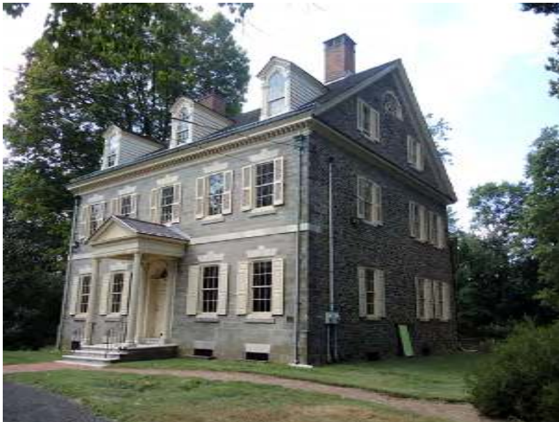
PHOTO 011 - Main Block, Northwest Corner (09-13-2016, NTHP)
