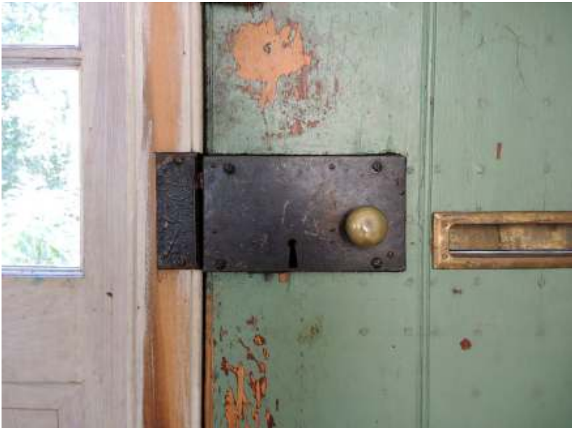
PHOTO 086 - Ell Interior, Room 106, Detail of Door Hardware (09-14-2016, NTHP)
