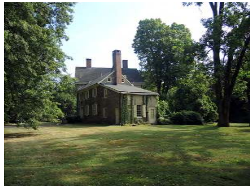
PHOTO 020 - Rear Extension, Southwest Corner (09-13-2016, NTHP)
