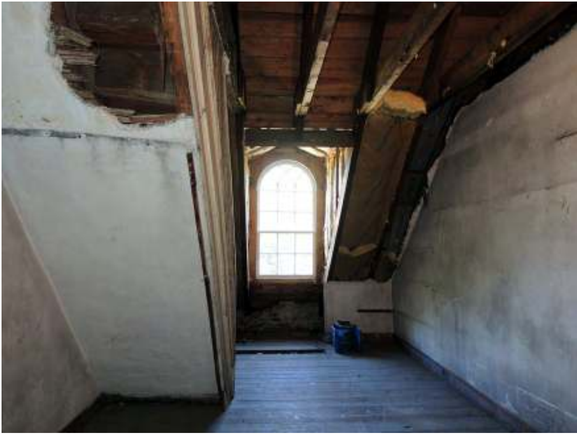
PHOTO 160 - Main Block Interior, Room 302, Looking Northeast (09-14-2016, NTHP)
